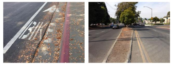
Figure 7: Northbound bike lane is narrow, with a seam between the pavement and gutter pan.
